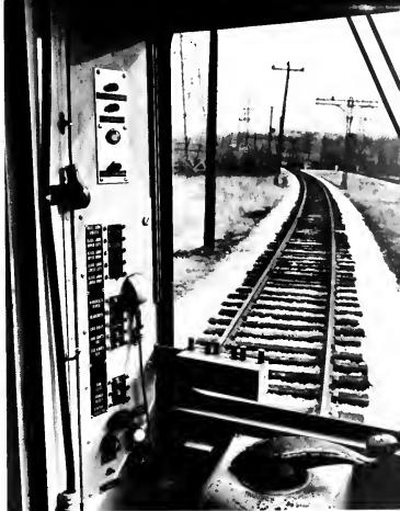
New panel of push buttons and pilot light at eye-height on operator's left provides complete control of pan trolleys.
